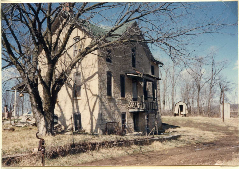
Back Kitchen door faces East. House as it appears Mar 1986
