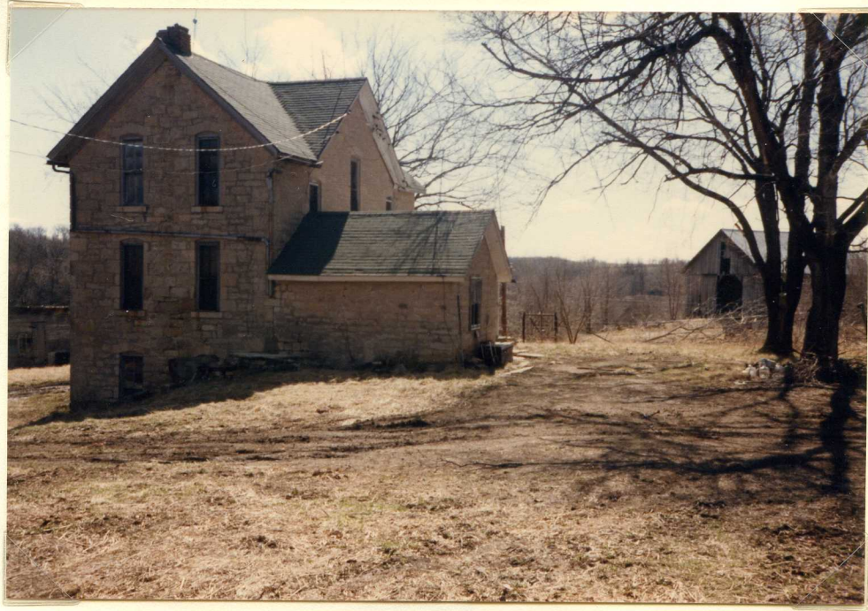
Hired hands' room add-on with root cellar under neath. Entrance to Cellar from Kitchen
